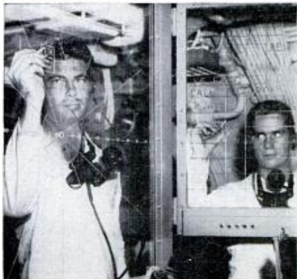
Evaluator in radar-picket sub directs U.S. planes to intercept enemy aircraft. Below, plotters spot positions of friendly and enemy planes on glass charts. Man at left is marking "TH" (target height)
